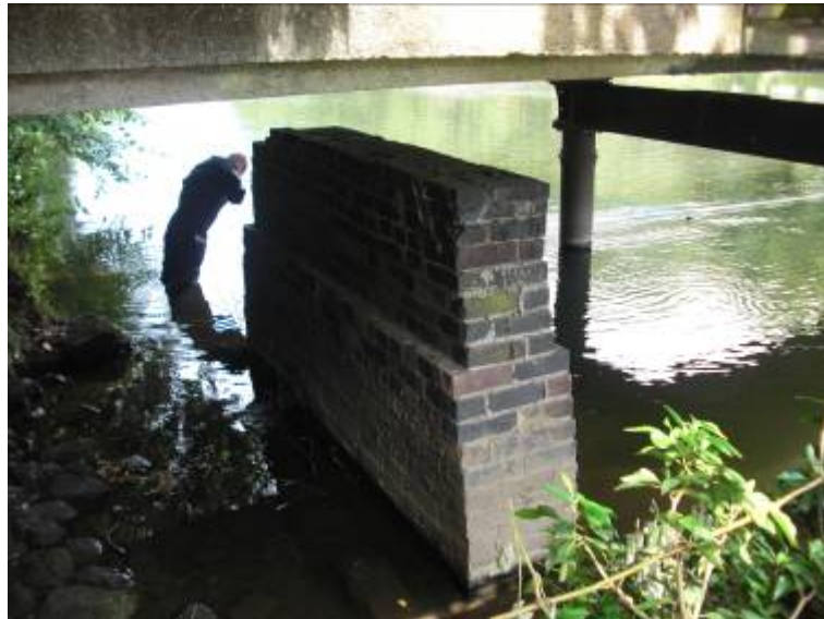
Picture 24 - Redundant brickwork / masonry pier between pier 5 and west abutment.
