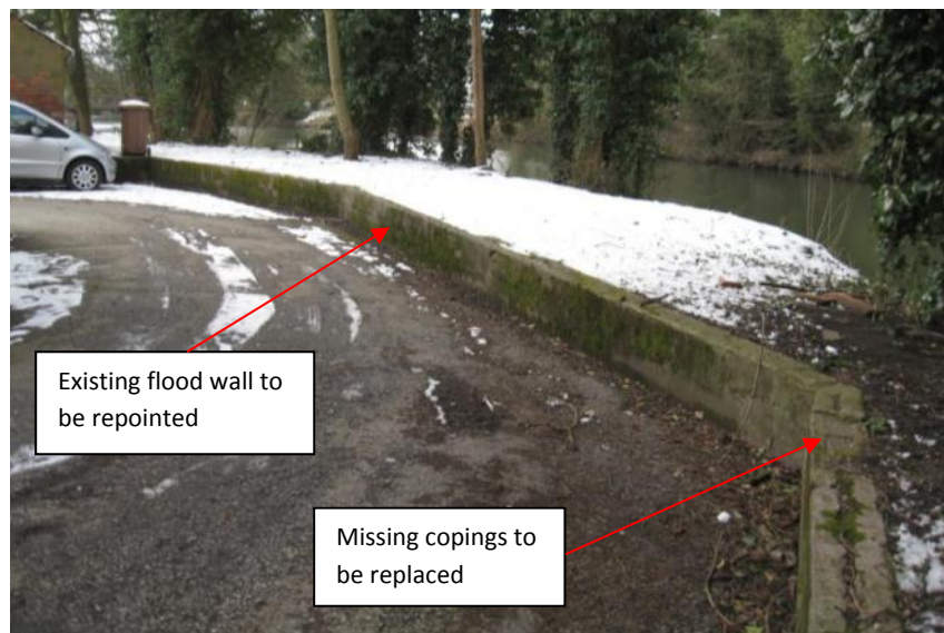
Figure 8.2: View of existing wall at Darley Abbey Mills to be maintained
