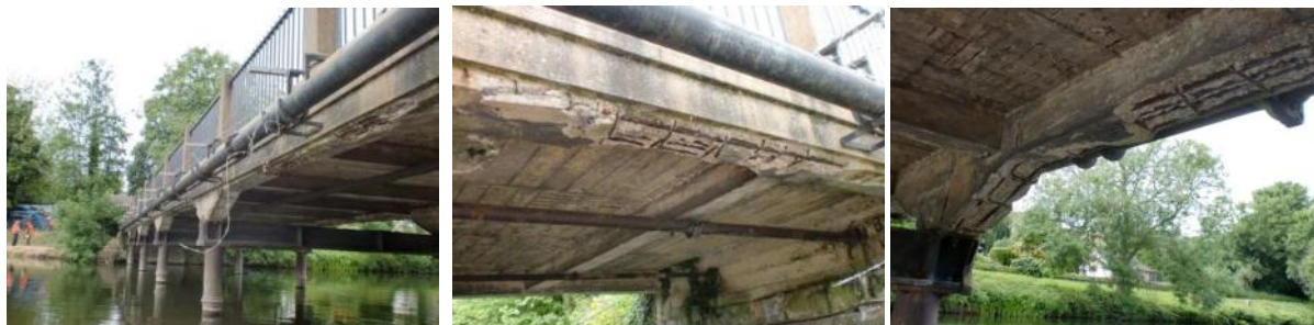
Figure 8.6: Existing condition of the underside of Darley Abbey Bridge
