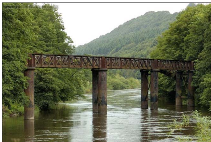
Figure 8.7: View of Redbrook railway bridge (Source: www.radnorimages.co.uk )
