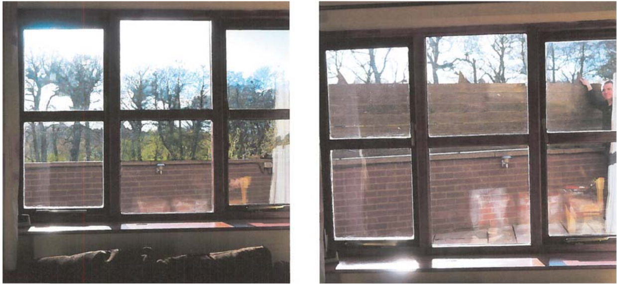
Figure 8.1: Views of existing flood defence and mock-up of raised defence from property at southern end of Folly Road.
